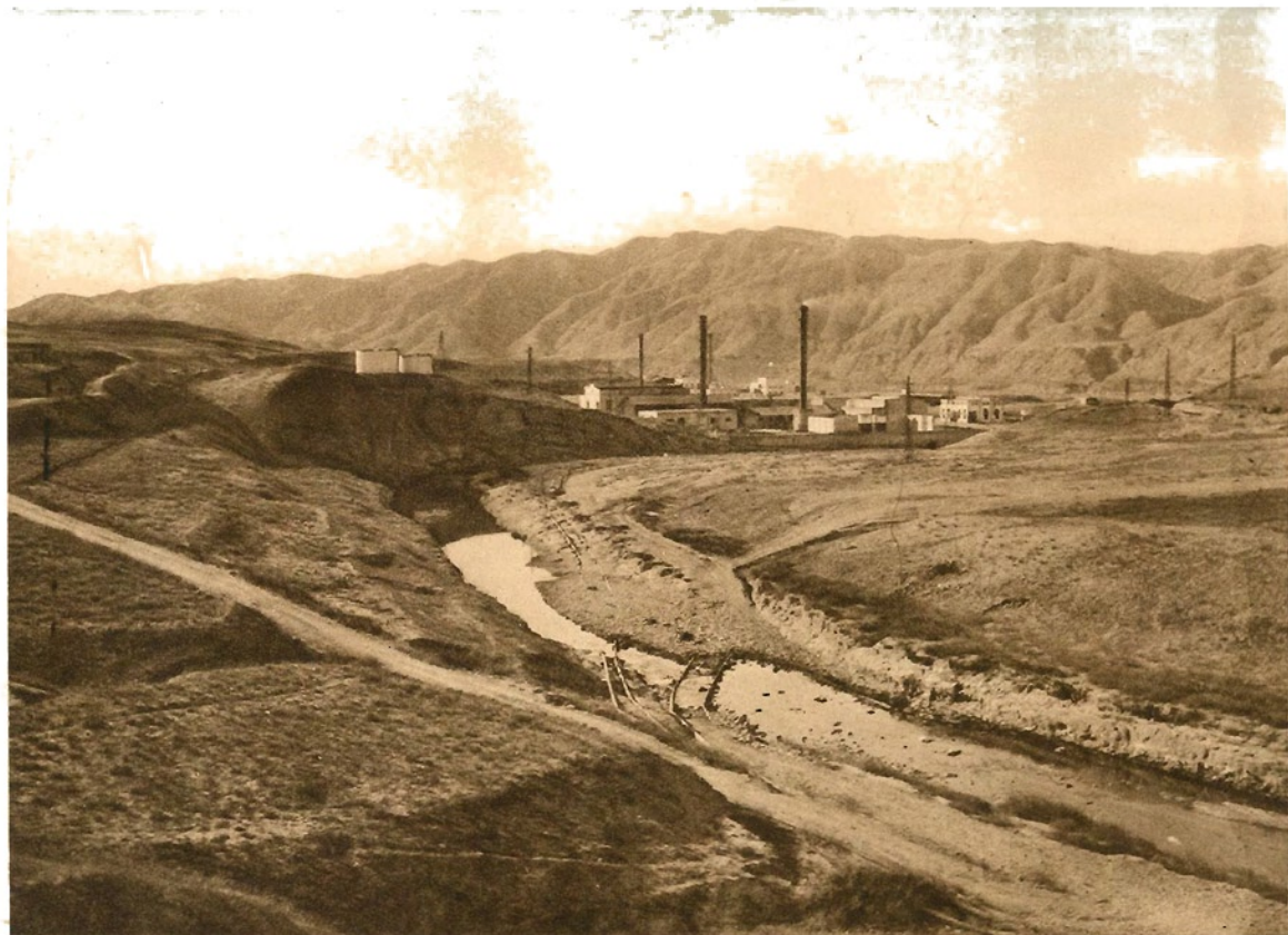
PUMPING STATION, TEMBI
