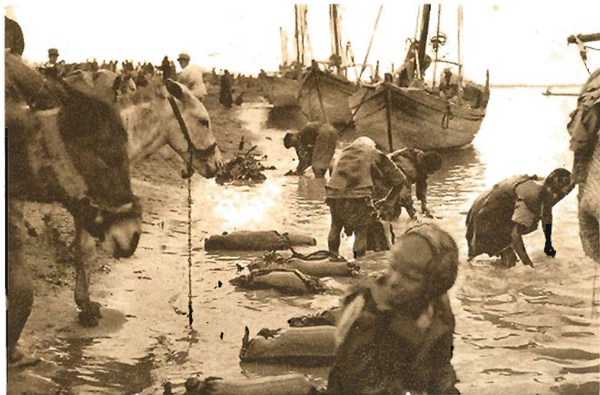
WATER CARRIERS. REPLENISHING SUPPLIES FROM THE KARUN RIVER
